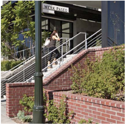
BRICK VENEER/ BRICK PATIO WALL
