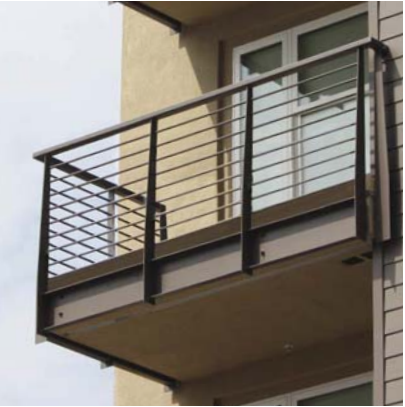
PAINTED METAL BALCONY RAILING
