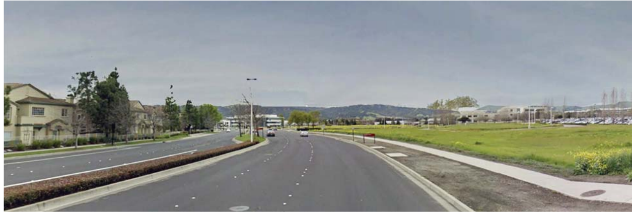
2. EXISTING VIEW SOUTH DOWN HACIENDA
